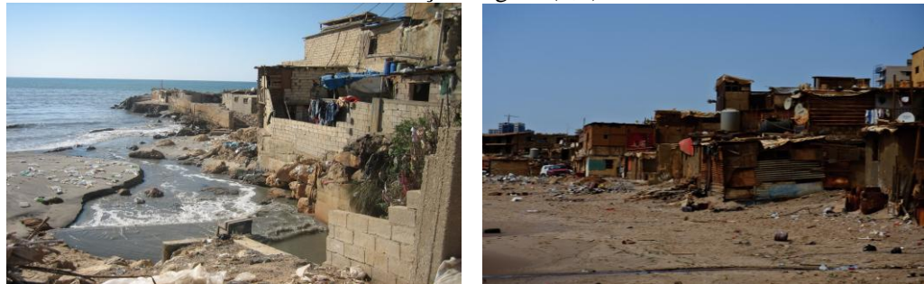
Figure 7, 8: Building quality in Ouzai Reference: Soubra, Lynn, The muted screams of Ouzai, World Press, Dec. 2012 https://lynnsoubra.wordpress.com/2012/12/16/the-muted-screams-of-ouzai/4005668468_65f3b1c469_b/
